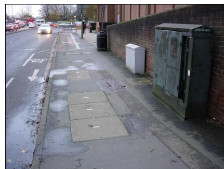
PHOTOGRAPH 6 EXISTING BT AND VIRGIN MEDIA CHAMBERS IN FOOTWAY ON THE CAUSEWAY (SOUTH SIDE)
