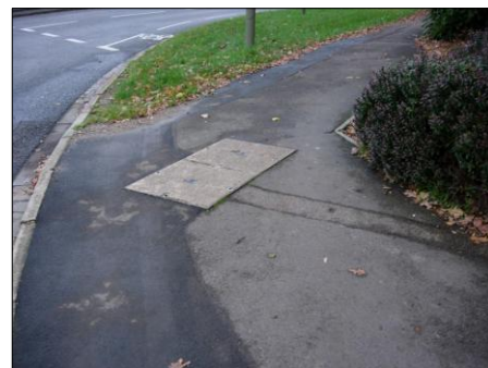
PHOTOGRAPH 3 EXISTING VODAFONE CHAMBER AND DUCT SCARRING AT JUNCTION OF THE CAUSEWAY WITH ACCESS ROAD
