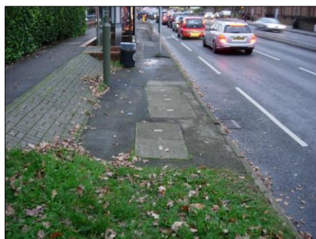
PHOTOGRAPH 4 EXISTING BT, VODAFONE AND VIRGIN MEDIA CHAMBERS IN FOOTWAY ON THE CAUSEWAY (NORTH SIDE)
