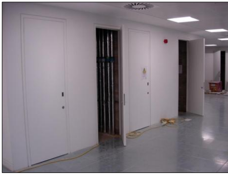
PHOTOGRAPH 10 TYPICAL RISERS ACROSS ALL FLOORS
